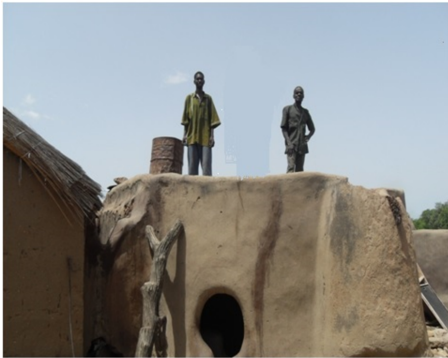
Fig.5 A photo showing how people were posted on roof tops to alert the community on the approach of slave raiders. Photo by the author.
