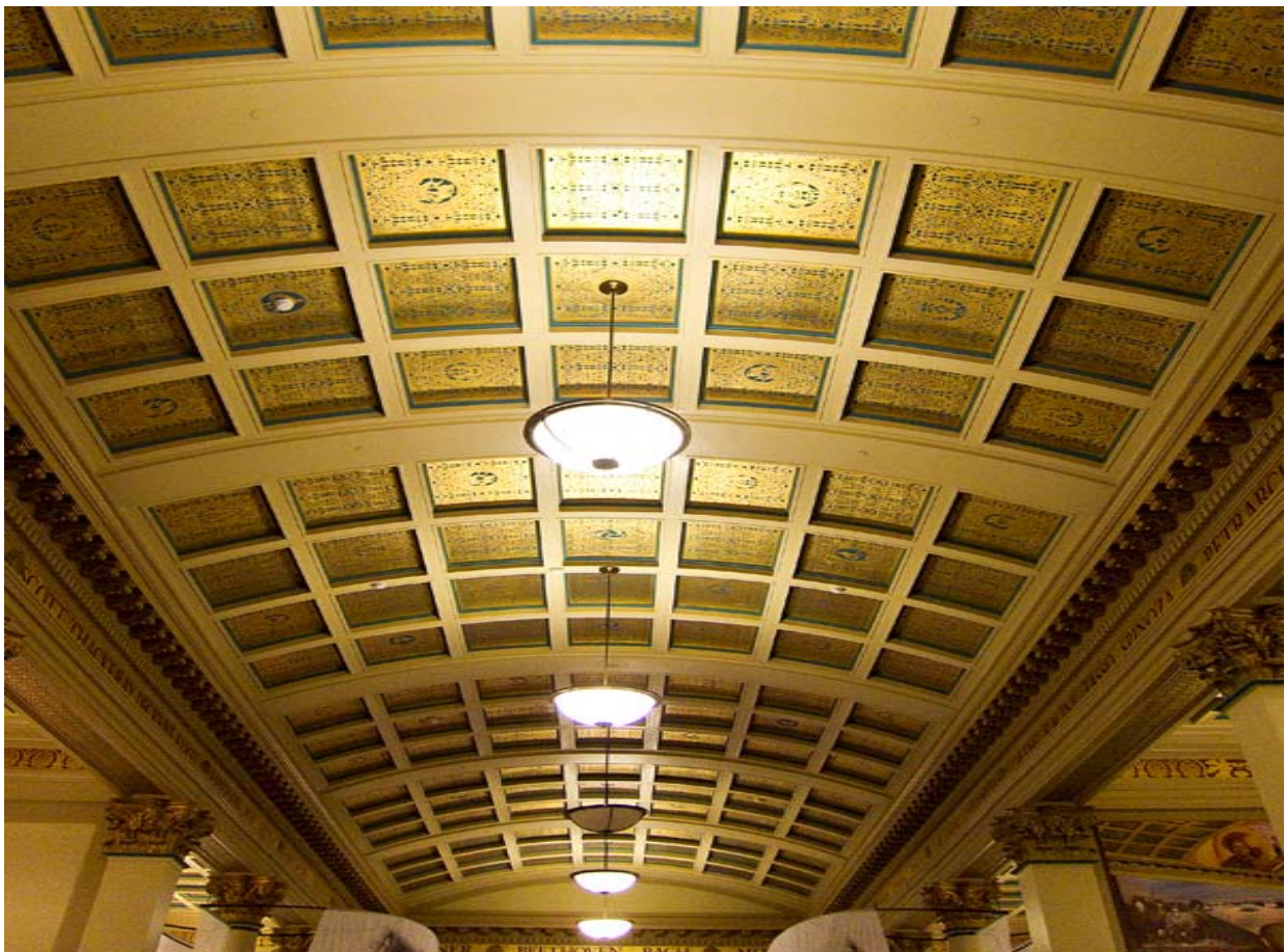
Ceiling architecture of the African American Museum and Library at Oakland
